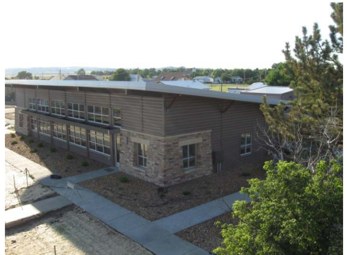
Landscaping finished. August 2011
