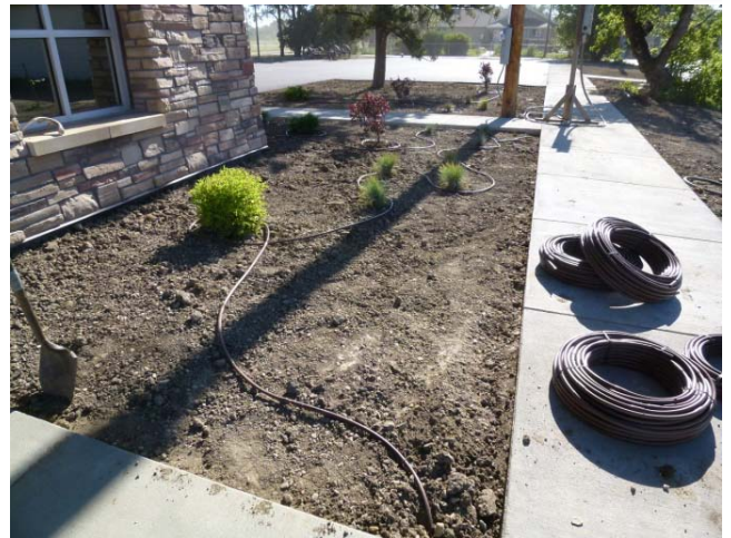
Drip line irrigation being installed for initial landscaping
