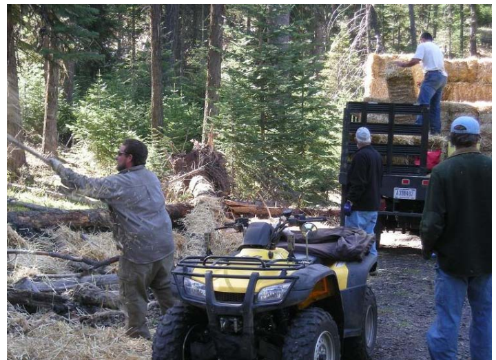
Working with partners to rehabilitate off-road damage.
