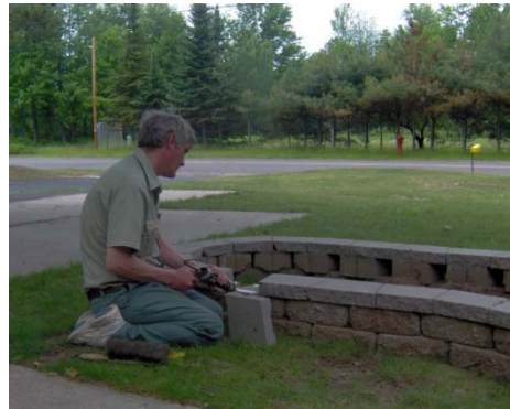
Figure 2. Retaining wall placed for shade garden at Ontonagon Ranger District
