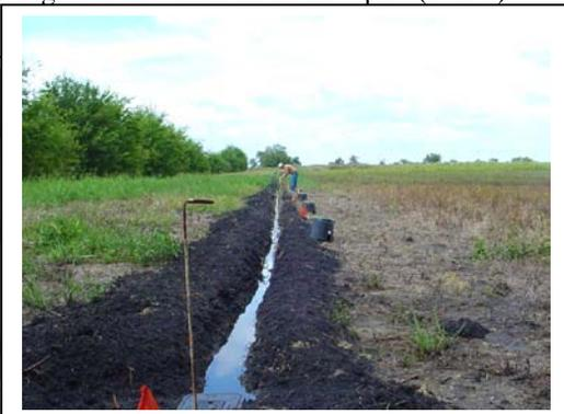
*More than 1,000 feet of buried irrigation line installed.*
