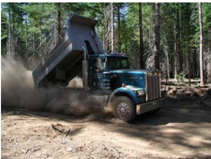
Laying biosolids on a soon-to-be farmed, greened-up, wildlife-enhanced storage road.
