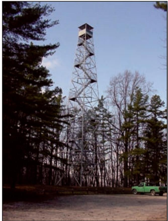
Figure 2—Steel towers may be coated with lead paint buried beneath many other layers of paint.
