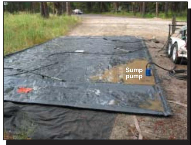
Figure 6—A 19- by 33-foot mat keeps the wash water where it can be recycled. Foam tubes are placed in slots along the mat’s edges to create a 3-inch lip on all sides. The mat shown here was set up at the Cathedral Fire near Darby, MT, during August 2002. The wash water drains to the lower right corner of the mat, where a sump pump draws water for filtering and reuse.
