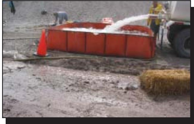
Figure 18—When vehicles are so muddy that it is impractical to reuse wash water, portable, soft-sided Fol-Da-Tanks could be used to store supply water and used water.
