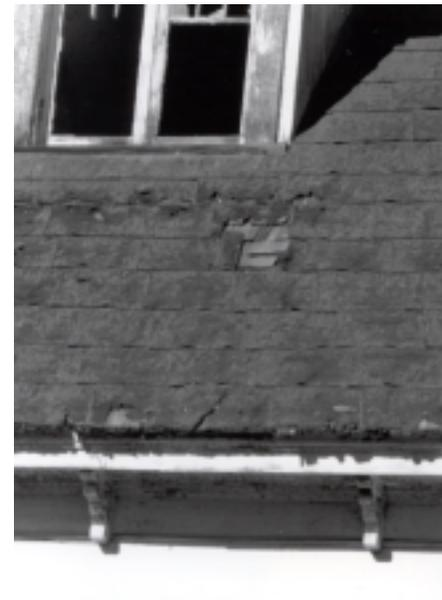
Figure 8—These old shingles are rotten, allowing the elements access to the building's interior.
