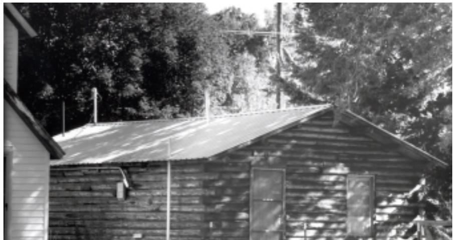
Figure 7—A log home with steel roofing.
