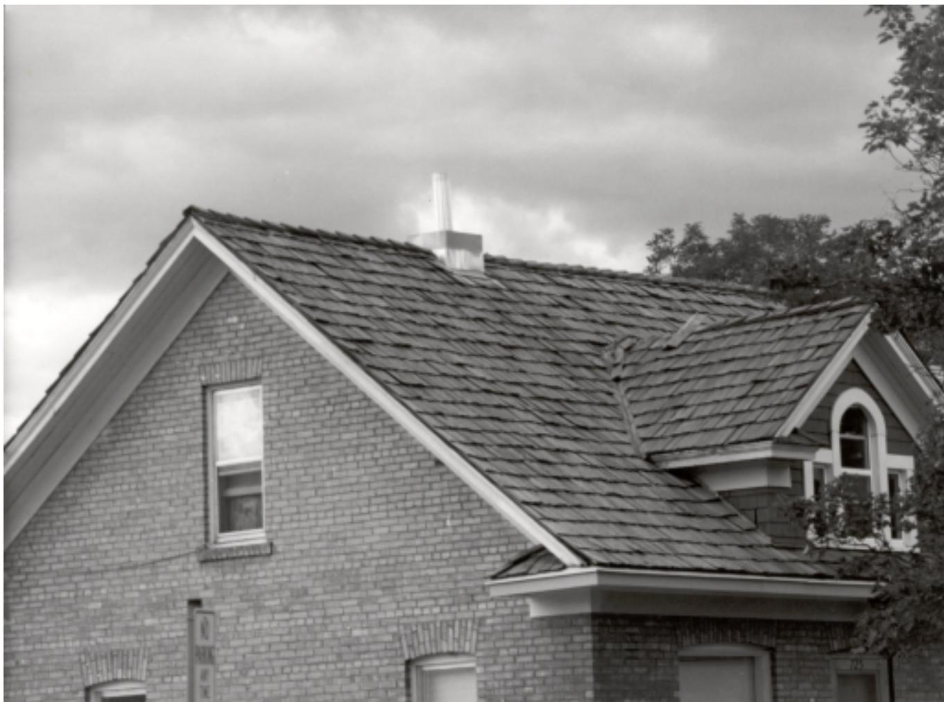
Figure 5—A wooden shake roof.
