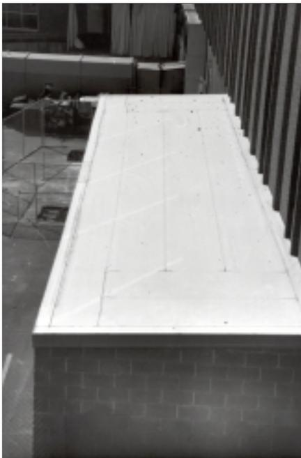
Figure 6—A low-sloped utility addition covered with a thermoplastic-resin roofing system.
