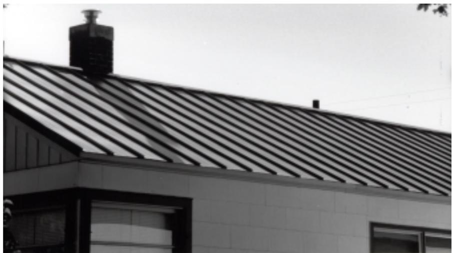
Figure 4—Metal roofing with a standing seam. The fasteners are under the seam.
