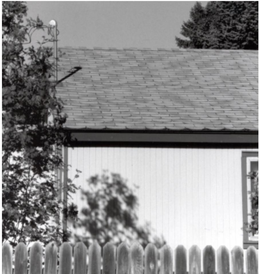
Figure 1—Residence roofed with asphalt shingles.
