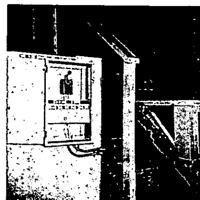
Figure 2.—View of stair lift and control panel is shown. When not in use, the lift platform is pulled up out of the way under winch at head of stairs, and rails fold up along far edge of stairway.
