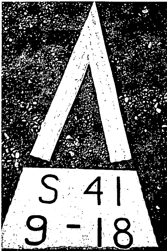
Figure 1.—A completed marker for a permanent helispot is shown.
