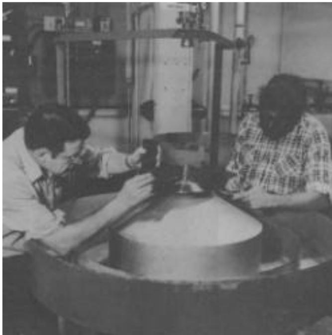
**An experimental spinning disk separator takes a stream of recycled paper slurry and spins sticky contaminate to an outer ring while dropping useable pulp fiber to an inner ring. (Credit: USDA Forest Products Laboratory)**
