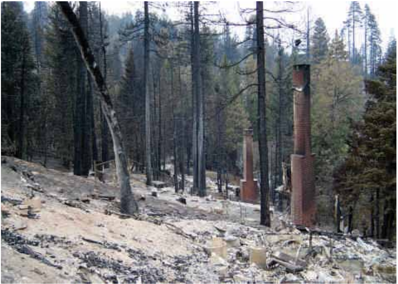
ABOVE: Unconsumed vegetation adjacent to four destroyed homes in this view indicates ignitions from lower intensity surface fires and/or firebrands directly igniting homes. • TOP RIGHT: This condition typically prevails across entire residential areas of WUI fire destruction. The areas of consumed canopy vegetation in this scene are related to homes burning. • BOTTOM RIGHT: High intensity fire spread in the tree canopy (crown fire) stopped at this residential street and did not continue as crown fire. However, all of the structures for several more blocks burned.
