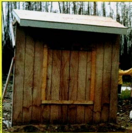
(a) 10-meter wood wall section before the crown fire.
