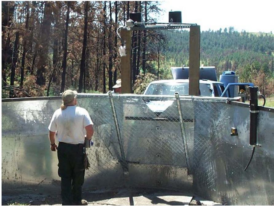
Figure 4. Large sediment basin and v-notch weir outlet
