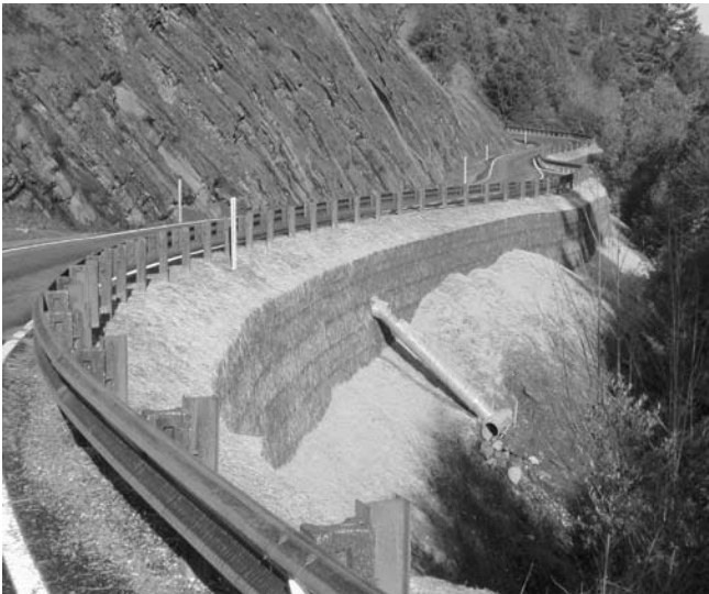
Figure 5 —In 2003, four months after gabion wall construction, seeded erosion mats were attached to the wire mesh at the face of the wall; compost amended soil was placed behind the screen and lightly tamped (A). Three years later (July 2006), the walls were fully vegetated and effectively screened from the road (B) (photos by David Steinfeld).
