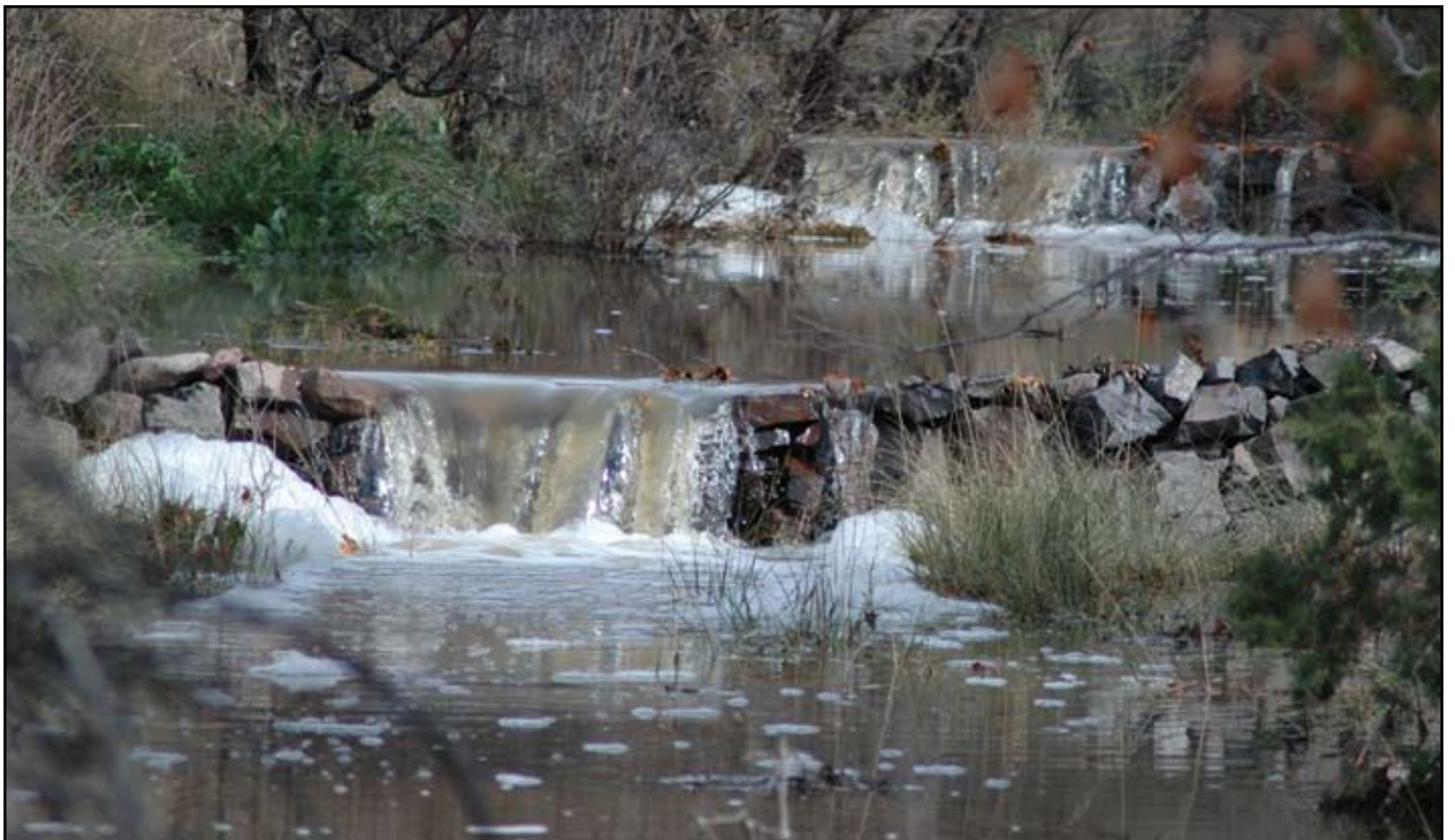
Loose rock structures withstanding flood waters.
