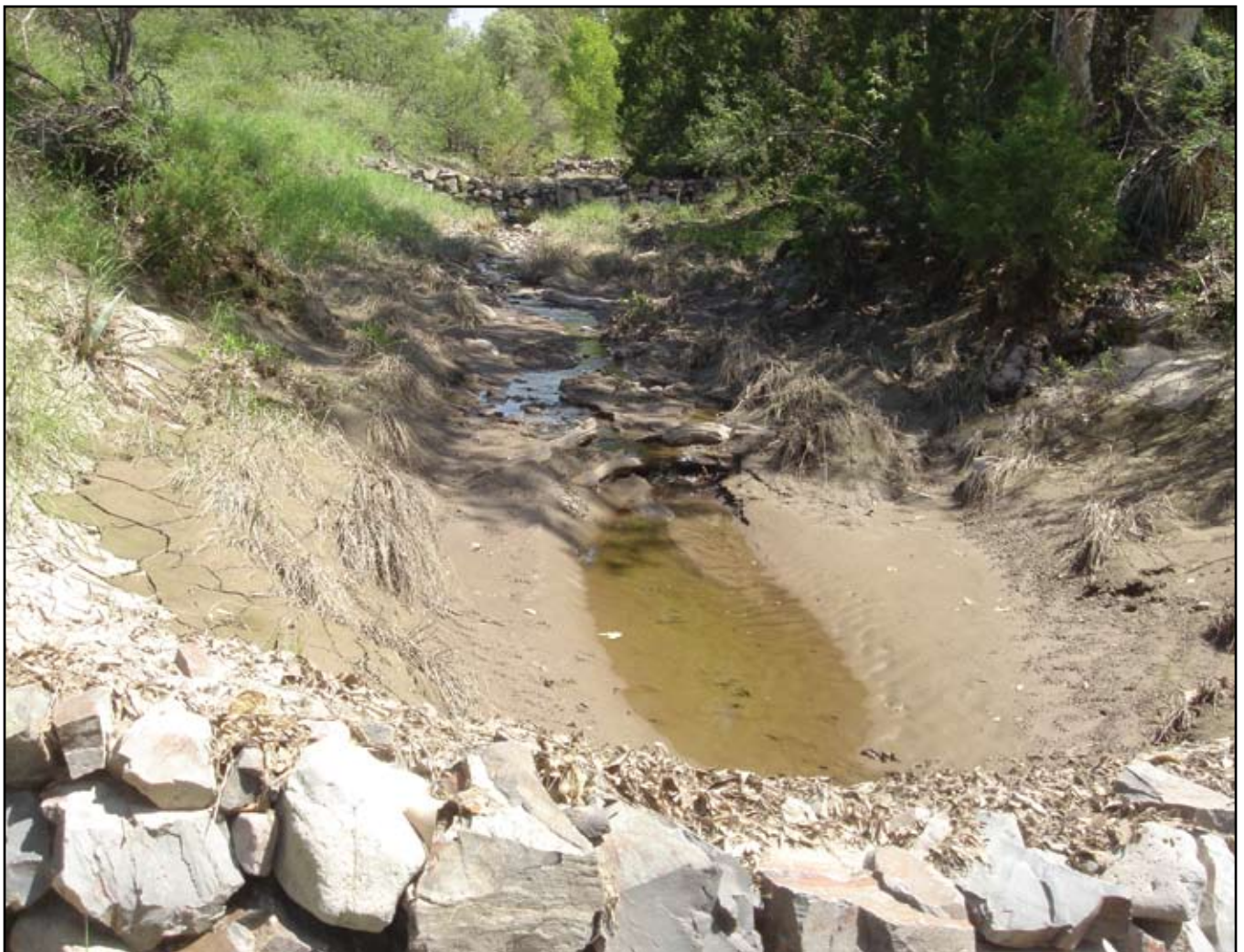
Loose rock structures constructed across streambed.
