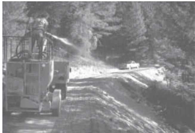
**Figure 33**—Hydroseeding roadcuts and fills.
