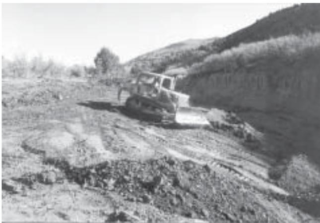
**Figure 36**—Three-way dozer reshaping a streambank.
