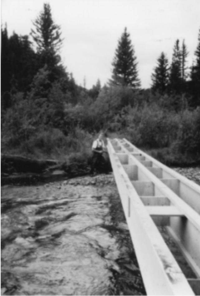
**Figure 5**—Plywood rectangles are used as spacers on this 3 x 60 foot platform on South Fork Cache la Poudre, near Fort Collins, CO.
