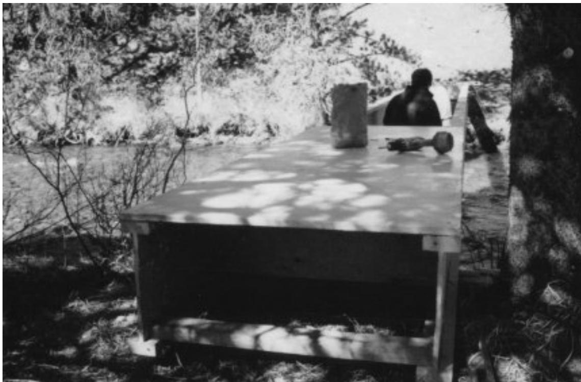
**Figure 10**—Plywood placed on a platform (3 x 40 feet) at Halfmoon Creek, near Leadville, CO. Note that the edges of the plywood are flush against the edges of the platform frame.
