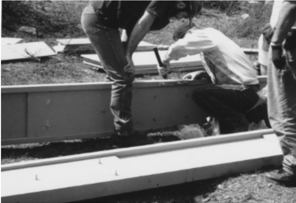
**Figure 8**—One of the 8 foot splices on a platform (2 x 48 feet) at Little Granite Creek near Jackson, WY. Note the metal plate (above the bent knee of the worker) used to add strength to the chord at the point where the two joists are joined.
