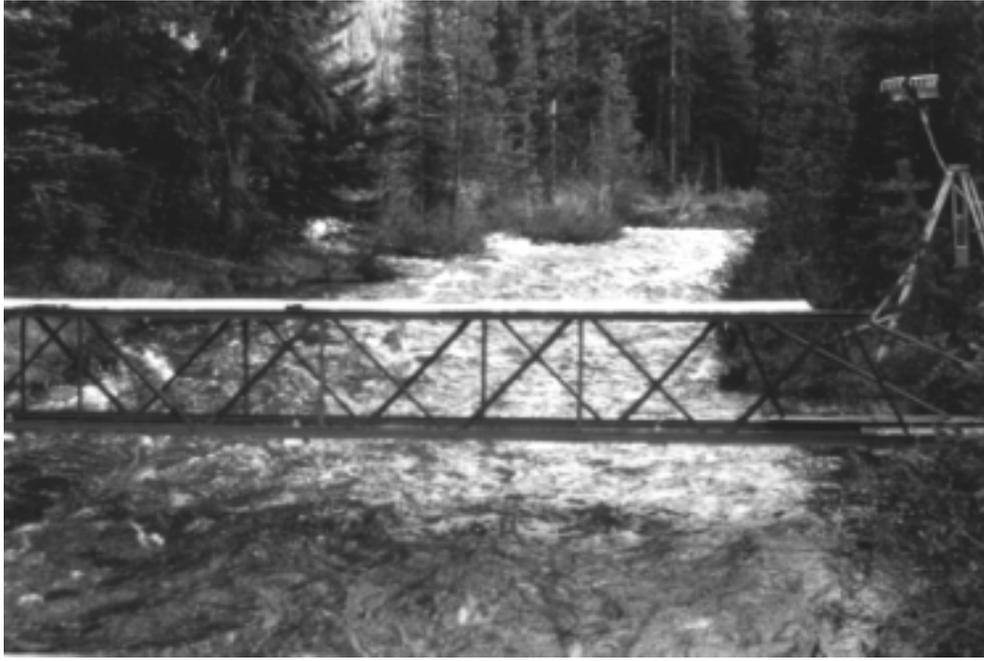
**Figure 1**—Platform constructed using steel bar joists at a site on St. Louis Creek, near Fraser, CO.
