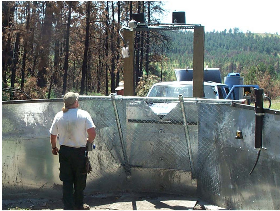
Figure 4. Large sediment basin and v-notch weir outlet
