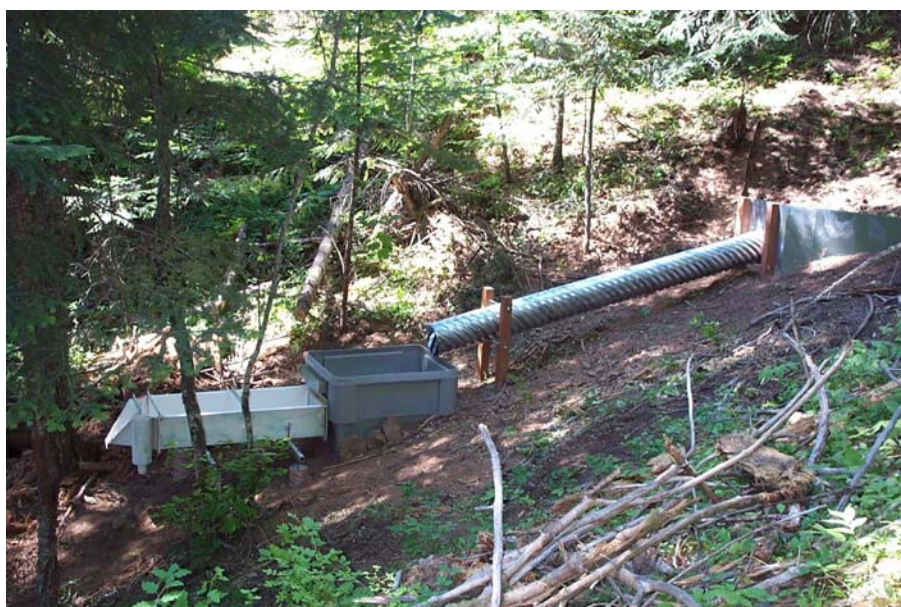
Figure 3. Collector, sediment basin, and h-flume on forested watershed.
