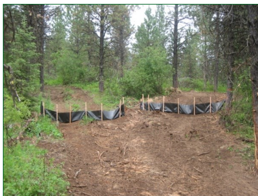
Silt fences used to study biomass impacts.
