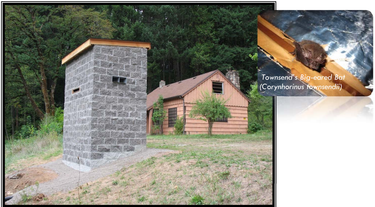
Hemlock Bat Bunker with West Hemlock House in background, which houses C. townsendii maternity colony.
