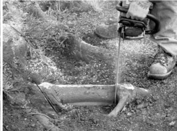
**Figure 2. Hand saws or chain saws with carbide blades are used for cleaner final cuts than obtained with the root pruning machine. Selective pruning of individual roots by hand is frequently performed prior to repouring sidewalks.**
