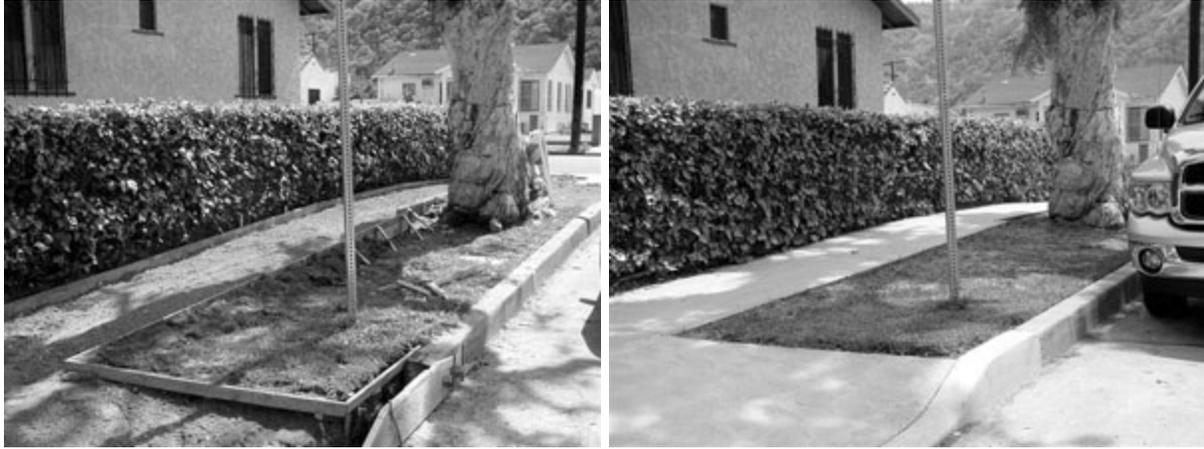
**Figure 4. Ramping the sidewalk reduces the amount of root pruning and is used to preserve highly valued trees. Ramping delays damage but does not provide a long-term solution to sidewalk heaving.**
