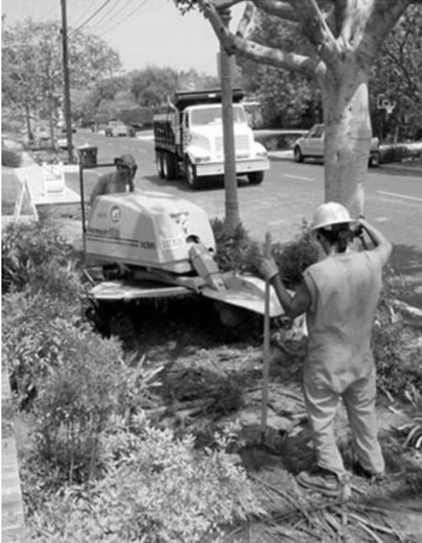
**Figure 1. Straight line root pruning is done initially with a machine through one quadrant of the root zone. The cut is made adjacent to the edge of the sidewalk and only as deep as needed for the sidewalk repour.**
