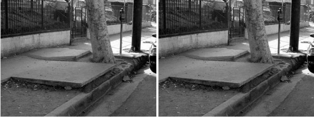
**Figure 3. Wherever possible, cut-outs are enlarged during the sidewalk repair process. In this case, the cut-out was enlarged parallel to the street so access for pedestrians was not impeded. Although not possible here, meandering the sidewalk around the tree increases the cut-out size, but requires permission from the adjacent property owner.**
