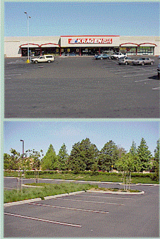
Photos of a parking lot before and after retrofitting.
