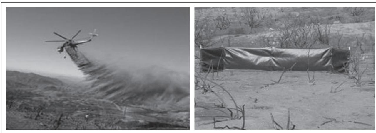
**Fig. 2.** Photos showing the aerial application of hydromulch at the base of Viejas Mountain and a constructed silt fence.
