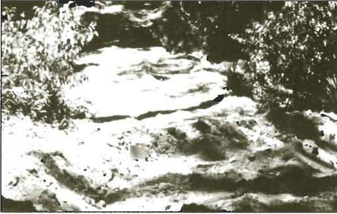
**Figure 1**—After logging, cross drains are provided on snig tracks to control runoff and prevent erosion on exposed soil surfaces.
