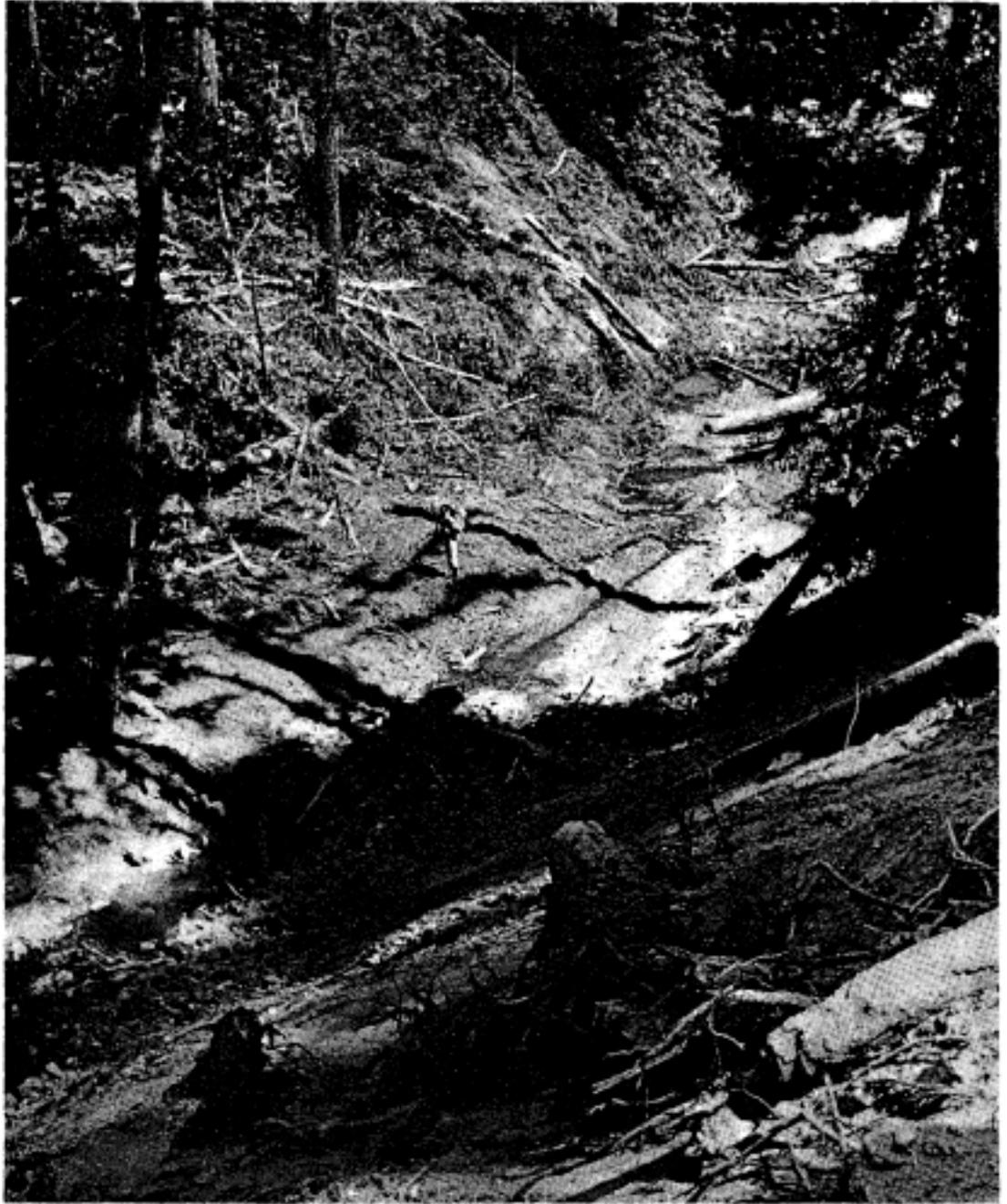
FIGURE 9.-South Fork Caspar Creek was grossly altered by road construction. The primary cause of damage was the operation of bulldozers in the stream channel.
