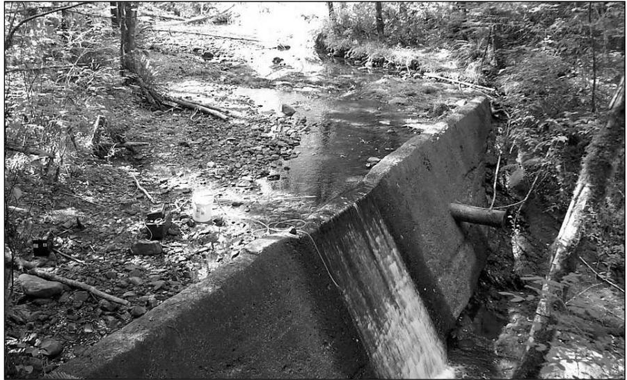
*The reservoir behind Dinner Creek Dam was completely full of sediment in 2002, before the dam was torn down. Photo by Greg Stewart.*
