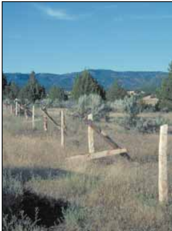
Photo 36—These juniper fence posts were made onsite by a rancher using a chain saw, Grant County.
