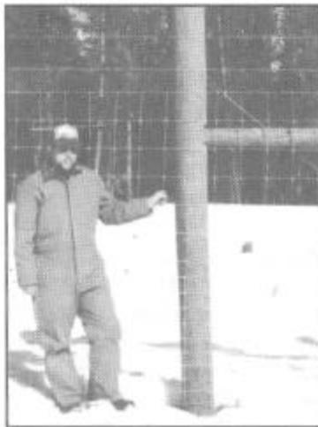
Figure 3—The Starkey fence encloses 25,000 acres and is 8 feet high, with two strands of smooth wire above the woven wire.
