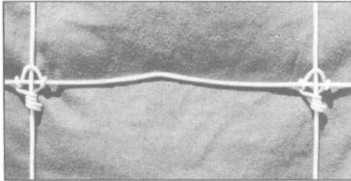
Figure 2—Tension curves and knots in Tightlock deer fence.
