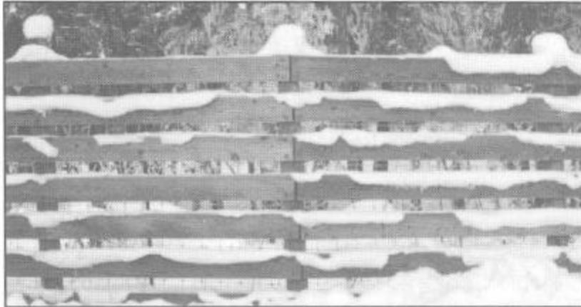
Figure 6—Boarded sections of the fence protect the Tightlock woven wire in areas of potential pressure from groups of elk.
