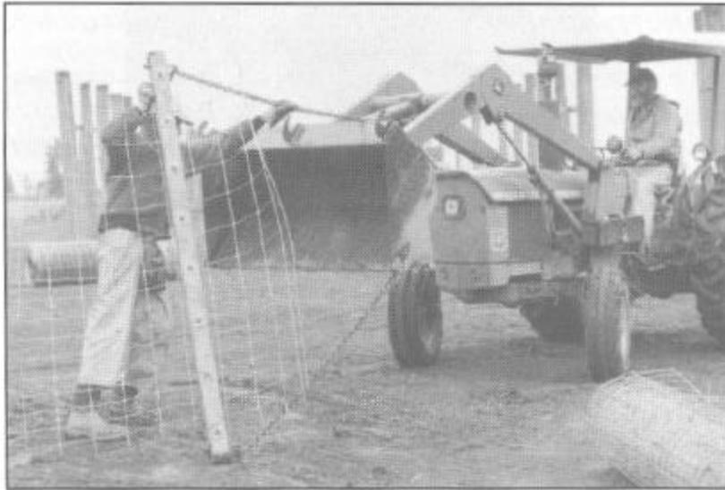
Figure 5—Stretching New Zealand woven wire with a strainer board attached to a tractor bucket.
