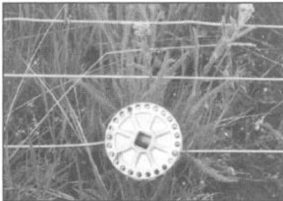
Figure 8—Rapid Wire tightener in place.
