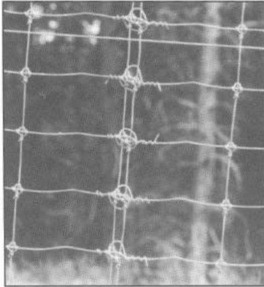
Figure 4—Spliced section of New Zealand Tightlock fence; note location of splice near vertical stays.
