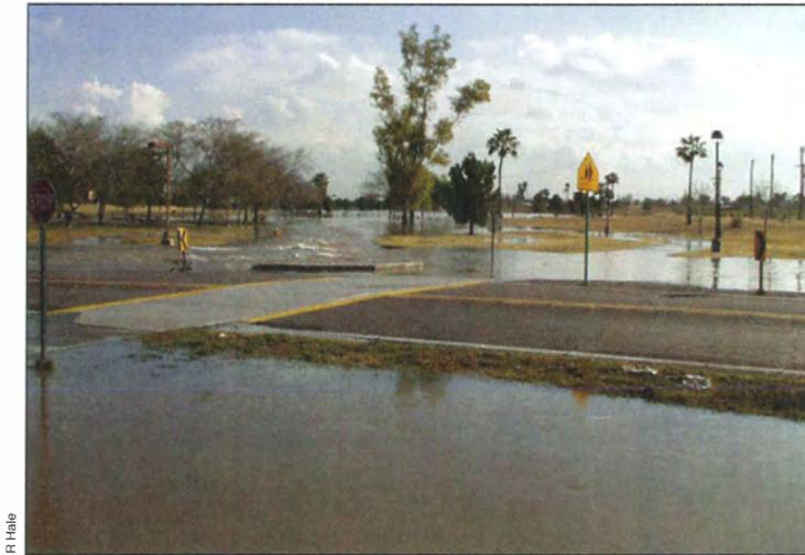
**Figure 2.** Indian Bend Wash, Scottsdale, Arizona, during a flood that covered a large portion of the “greenway”, which spread out over parks, golf courses, and streets, but resulted in minimal damage. This design was one of the first non-structural flood management systems in the US, created by local and federal government officials after damaging floods occurred in the 1960s.
