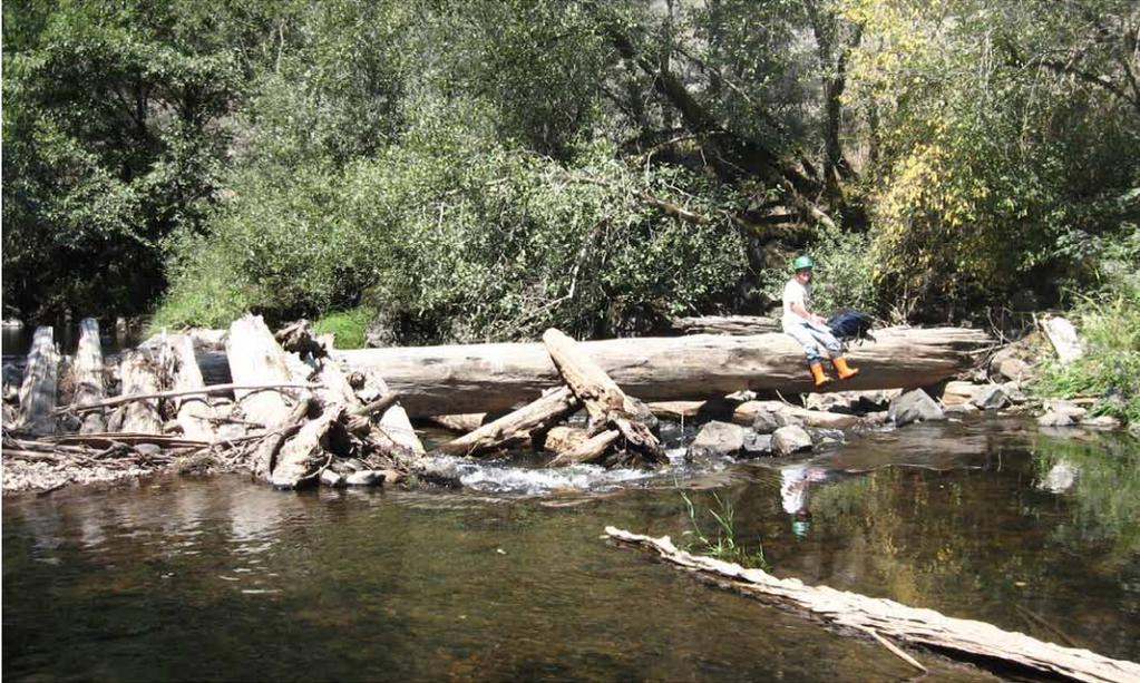
**Figure 4.** The Little Fall Creek splash dam was the most intact structure found during searches. Splash-dam cribbing and boards are still present. Remnant is approximately 12 m across, 1.5 m high, and structural cribbing extends 20 m downstream; note notched spillway (center) allows for fish passage. Photograph taken in 2009 by R. Danehy.
