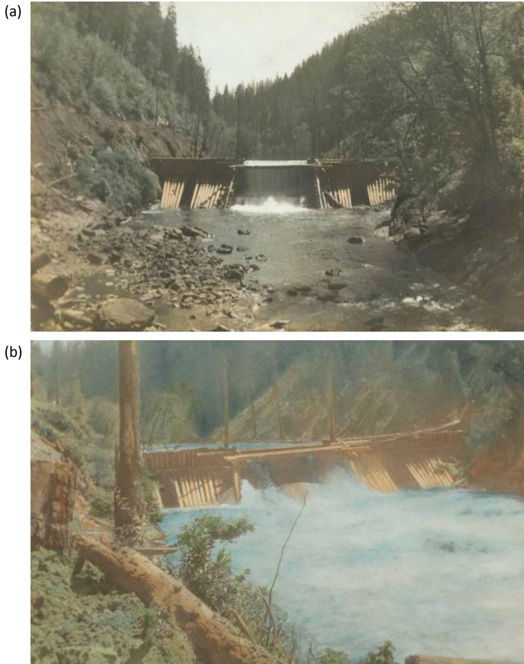
**Figure 1.** Upper dam on the South Fork Coos River, circa 1947. Length, 256 feet, height, 40 feet, it was built by the Irwin & Lyons Logging Company. (a) Closed. (b) Opening. Photos courtesy of Jake Flitcroft.
