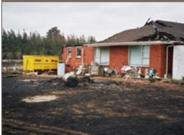
FIGURE 2. The fire resulted in significant damage—grasslands, wood lots, orchards, a vineyard, outbuildings, hedges and fences, farm equipment and a house were destroyed over an area of 130 ha.
