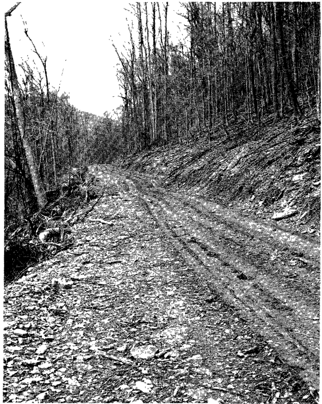
Figure 1.—A minimum-standard road section with a broad-based dip.
