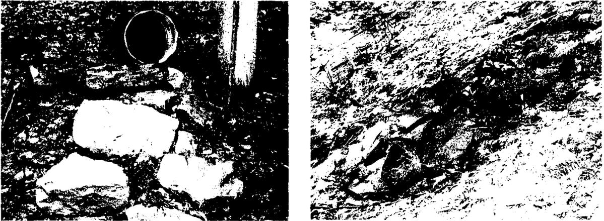
Figure 2. Examples of improper stair-step stacking (left) and layering of rock for erosion control (right). Rocks should be positioned as irregularly as possible to provide maximum roughness for energy dissipation.
