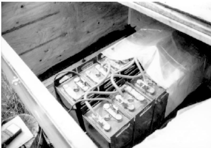
Figure 5—Storing batteries in the ground isn't recommended...
