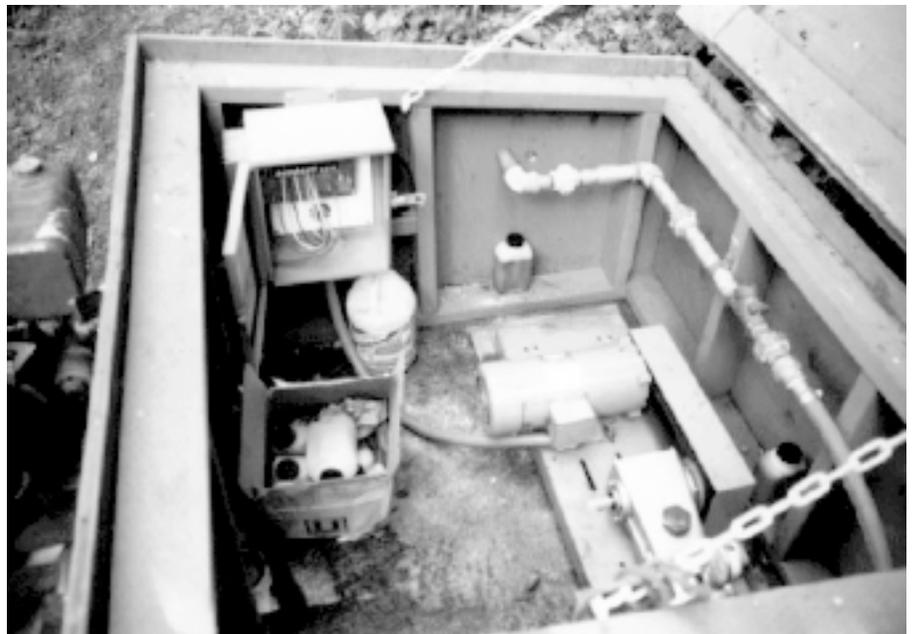
Figure 4—A photovoltaic-powered water pump installation at Wade Lake Campground on the Beaverhead National Forest in Montana.
