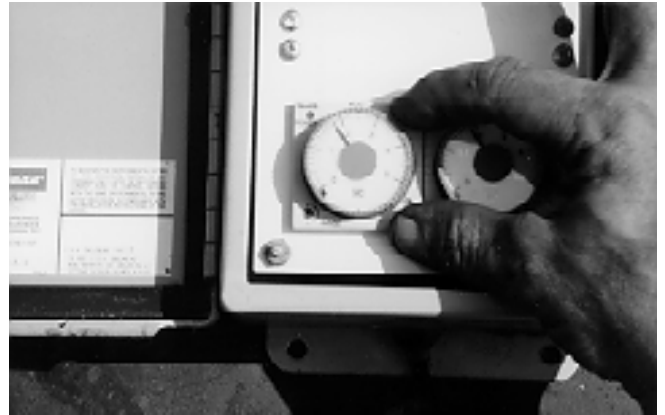
Figure 18—Adjusting the air solenoid timer.
