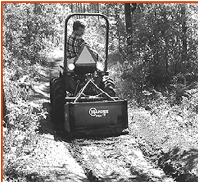
Figure 25—This box scraper, cut down to a width of 3 feet (0.9 m), does a good job of removing whoop-de-dos, but requires a skilled operator and a tractor.
