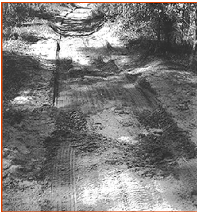
Figure 12—In the South Carolina demonstration, the Ultra Light Terrain Grader was very effective in removing whoop-de-does after several passes down the trail.
