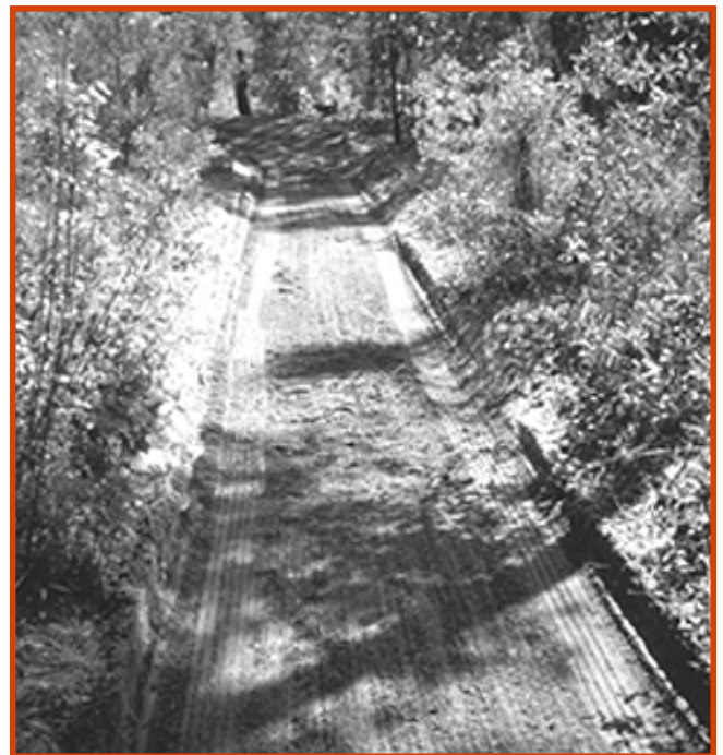
Figure 12—In the South Carolina demonstration, the Ultra Light Terrain Grader was very effective in removing whoop-de-does after several passes down the trail.
