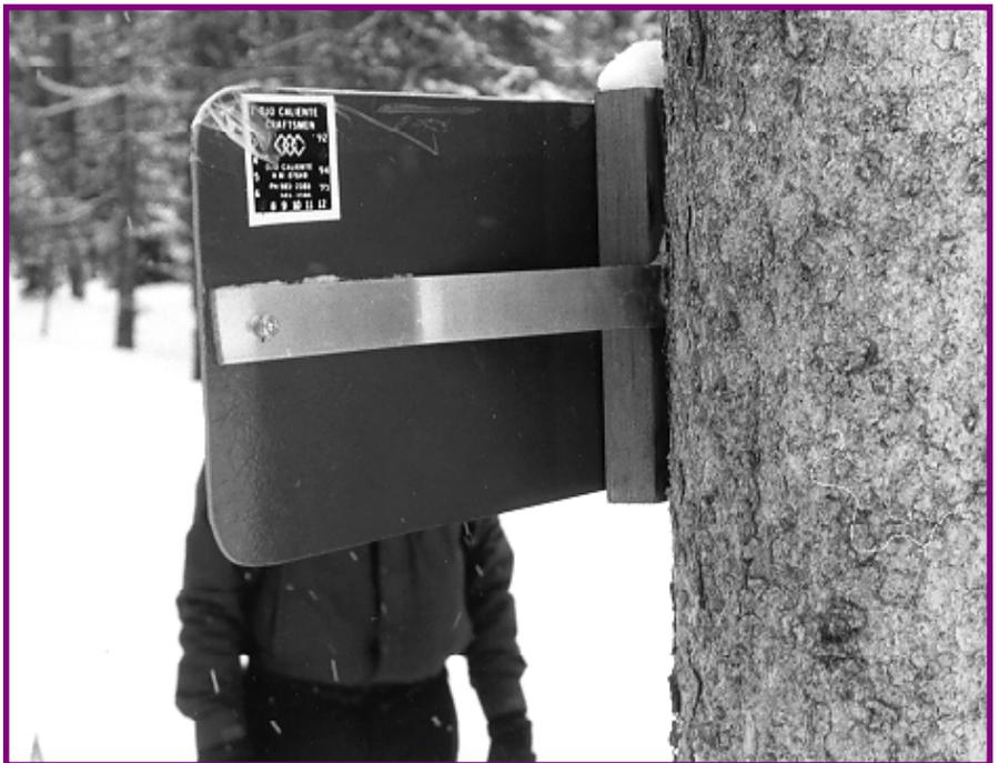
Figure 6—Metal braces can strengthen sign supports on larger signs.
