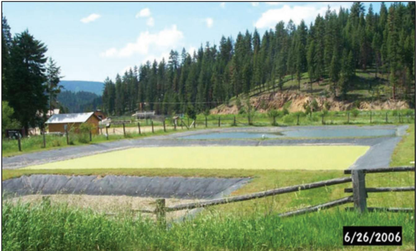
Figure 1—In June 2006, the second cell (bright yellowish green) of the wastewater lagoon at the Red River Ranger Station near Elk City, ID, was choked with duckweed. Triploid grass carp were released into the lagoon later that month.
