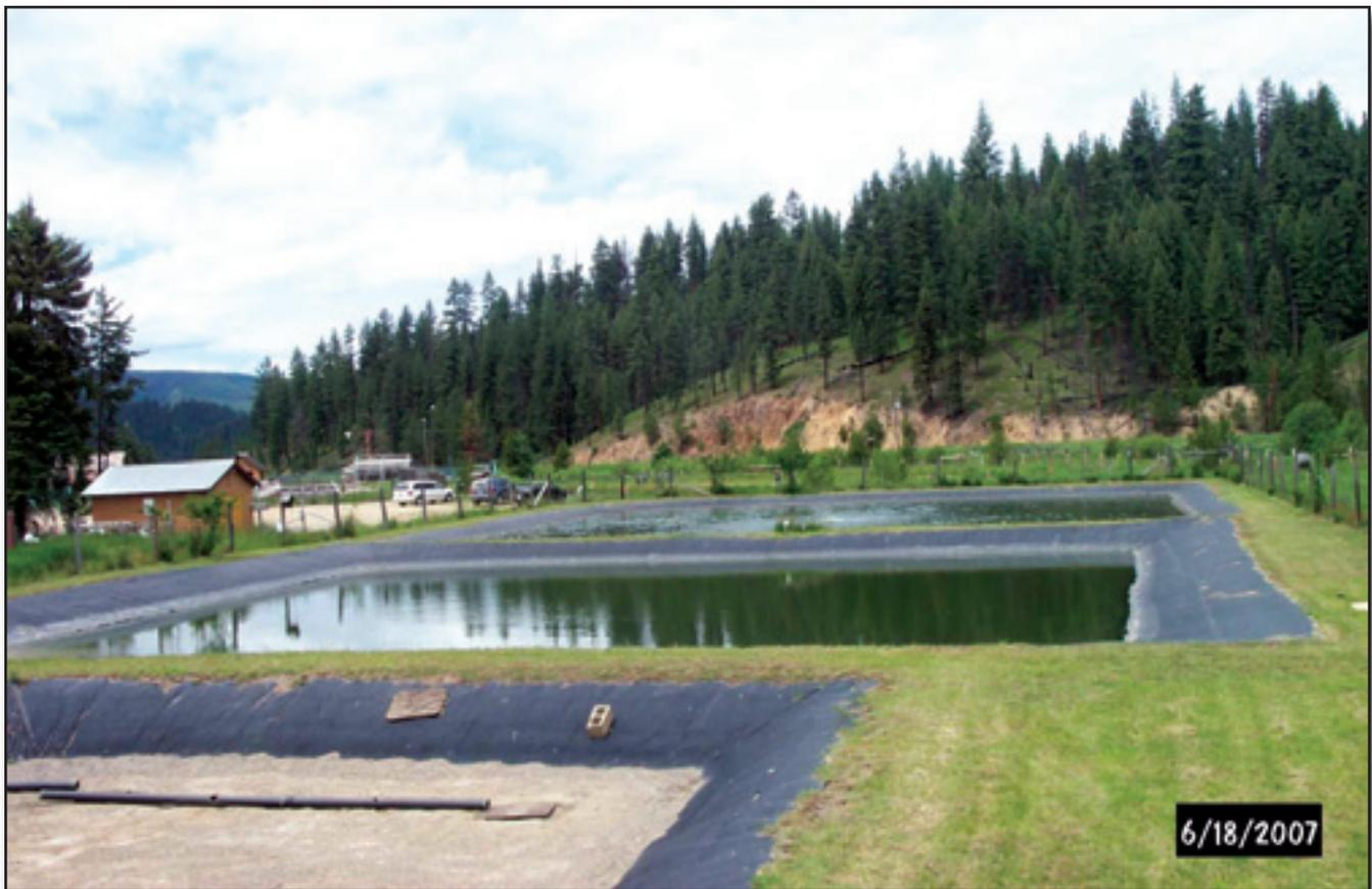
Figure 2—By June 2007, the triploid grass carp had almost completely eliminated the duckweed in the Red River wastewater lagoon.
