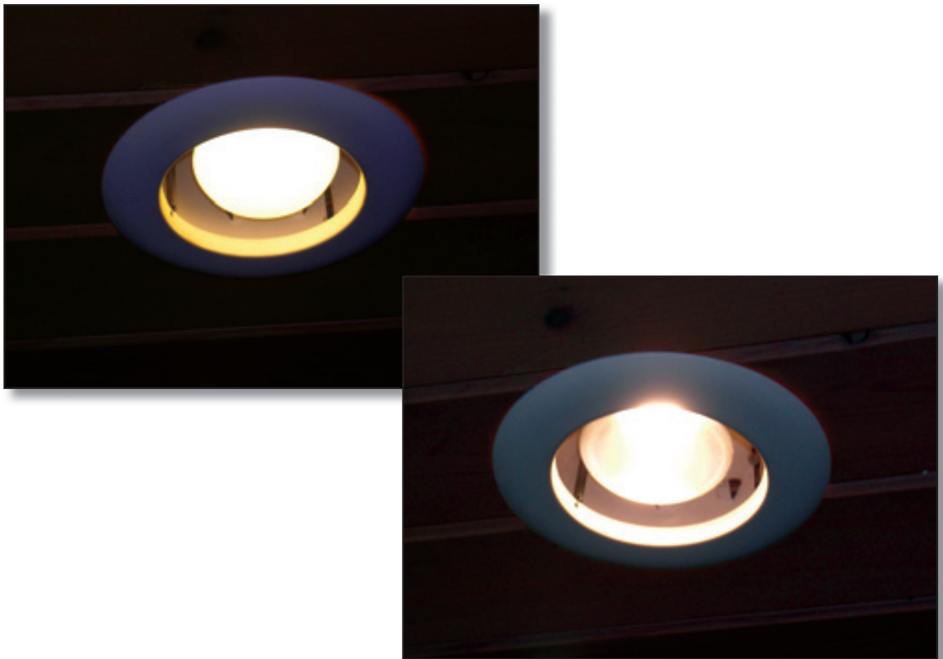
Figure 1—A 16-watt CFL floodlight on the left. A 65-watt incandescent floodlight on the right.
