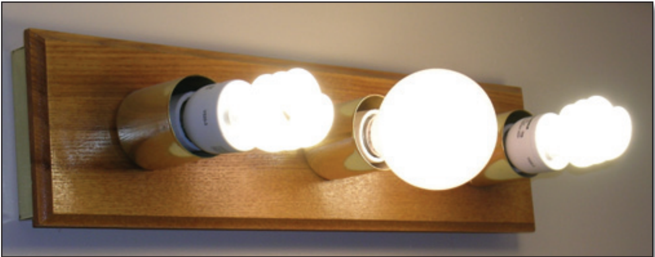
Figure 6—A vanity light fixture with one incandescent light bulb and two CFLs. The incandescent bulb will provide light while the two CFLs are warming up.
