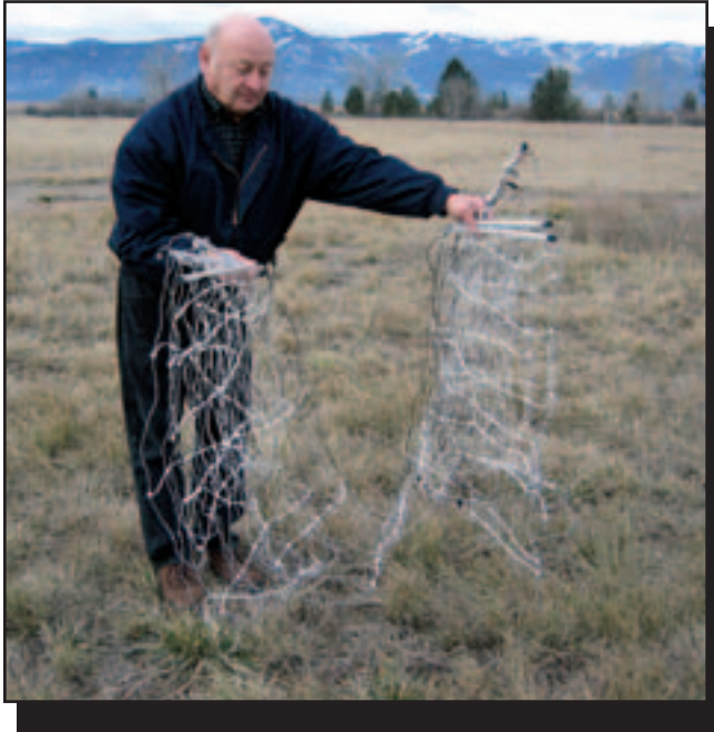
Figure 7—If the fence mesh has been gathered accordion style, the fence will be easy to install.
