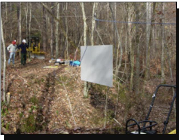
Figure 12—A skyline system can be used to haul bridge materials to an abutment across a stream.
