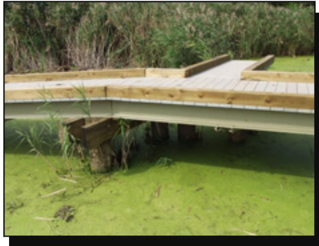
Figure 6—This boardwalk on Staten Island was constructed using an FRP deck-beam system.—Courtesy of E.T. Techtonics, Inc.
