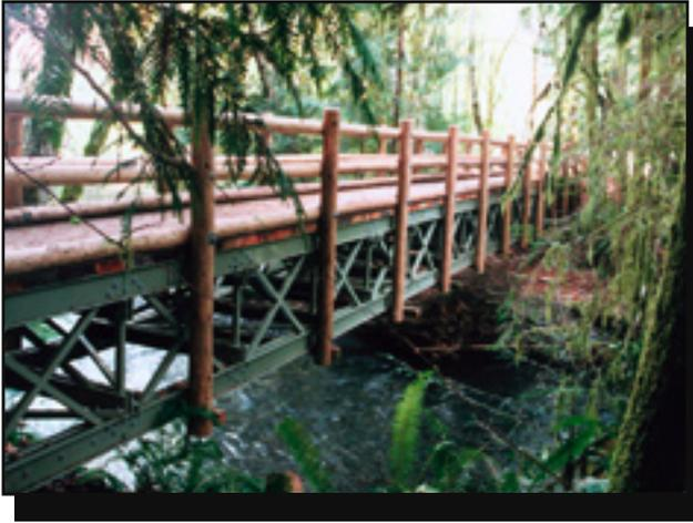
Figure 7—A deck-truss FRP bridge in Olympic National Park. This bridge uses FRP materials for the trusses and wood for the rails, maintaining a natural appearance for a high-tech structure.
