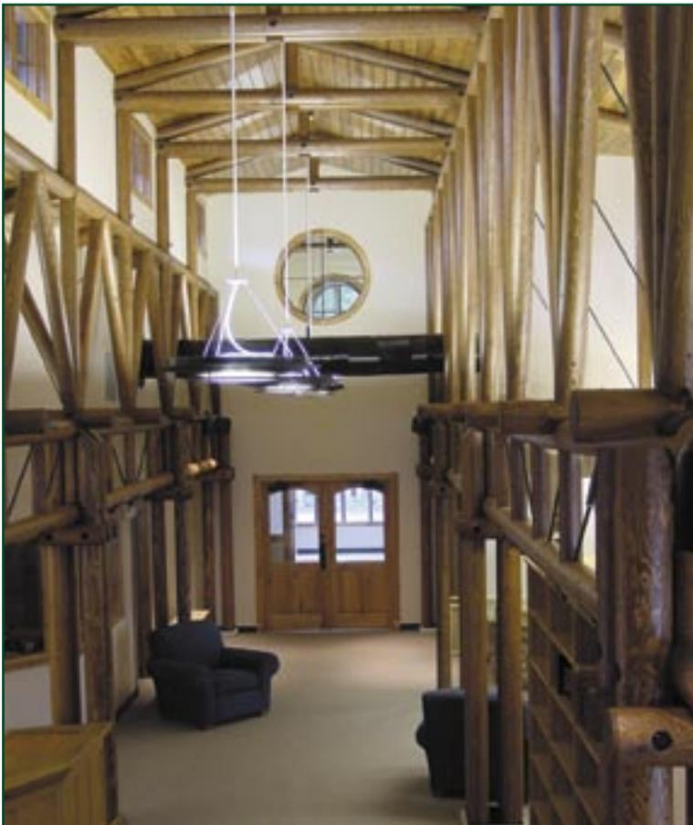
Figure 1—Interior of the new library in Darby, MT, that uses small-diameter roundwood.
