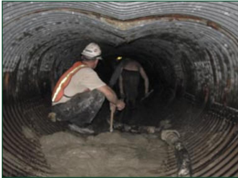
Figure 8—Grouting the old pipe. Note its condition.
