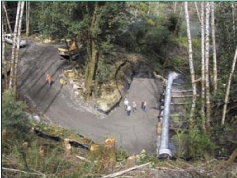
Figure 1—View from the road: the stream bypass pipe, the access road, and the launch pad.
