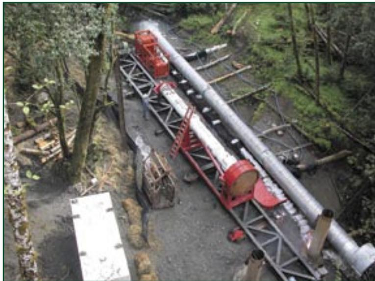
Figure 4—This view shows the operation from the other side of Quosatana Creek. The green vibratory pile hammer is suspended from the crane as it drives pipe piles.
