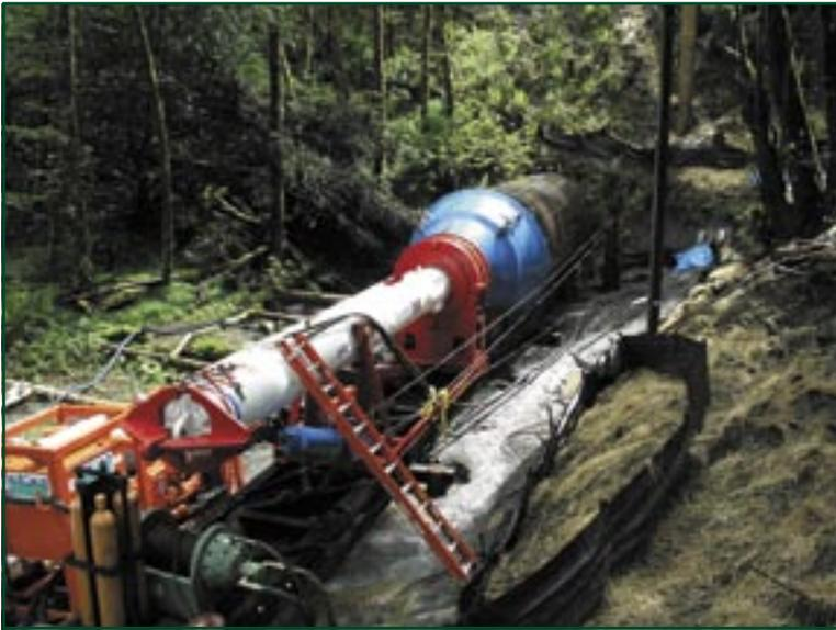
Figure 5—The hammer setup is complete. The first pipe section is in place before driving starts.
