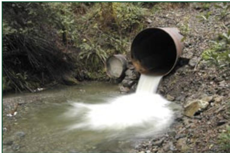
Figure 10—The new pipe's outlet. The grouted old pipe is to the left.
