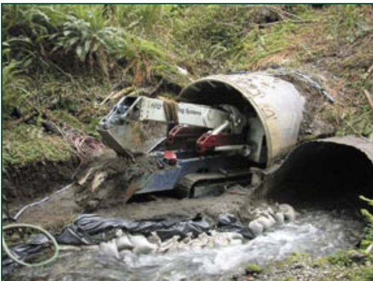
Figure 7—A tunnel excavator completes the job of cleaning out the new casting. It scoops up soil onto a belt between its tracks and transports the soil to the other end of the casing where the soil is loaded onto a truck.
