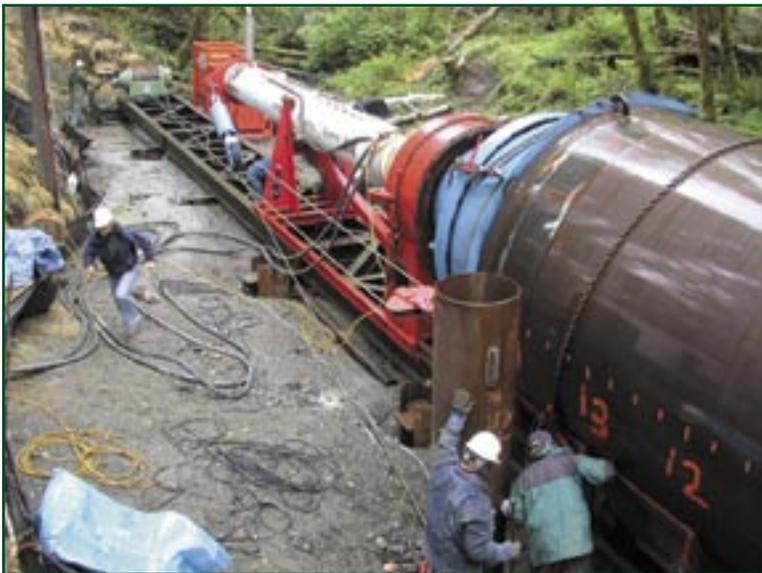
Figure 6—The hammer in action. The casing, shoe, helmet, and hammer are in place on the track. The winch is set up at the end of the track and takes up the slack in the system between hammer blows.
