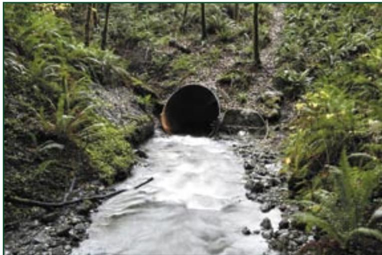
Figure 9—The new pipe's inlet. The grouted old pipe is just to the right.
