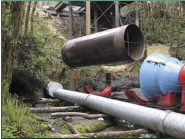
Figure 3—The first section of casing is being lowered onto the cradle with the crane. The blue cone at the right is the shoe, which transfers force from the hammer to the casing.
