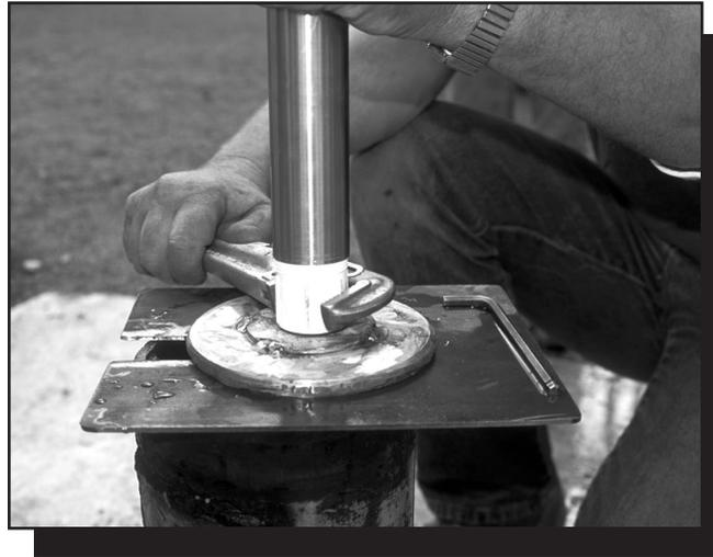
Figure 3—The accessible handpump is easily installed on standard well casings.
