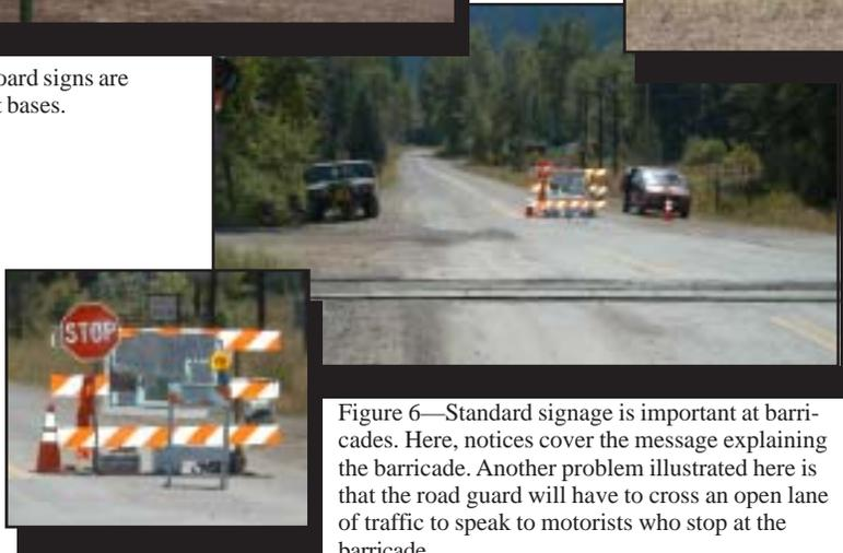
Figure 6—Standard signage is important at barricades. Here, notices cover the message explaining the barricade. Another problem illustrated here is that the road guard will have to cross an open lane of traffic to speak to motorists who stop at the barricade.
