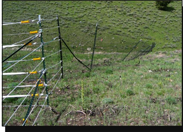
Figure 18—This plastic fence and support posts were probably bent over by a melting snow bank.
