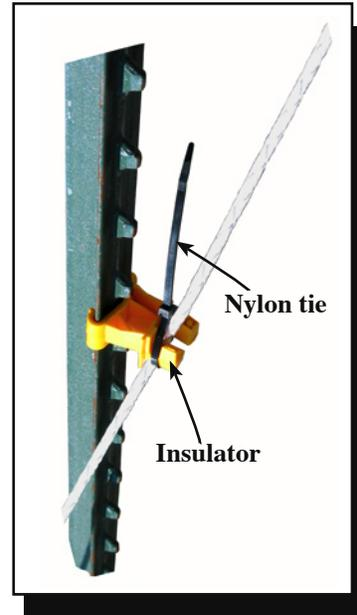
Figure 17— After wind or snow forced the polyrope out of its slot on the T-post insulator, grounding the fence, we used nylon ties to secure the rope to the insulator.
