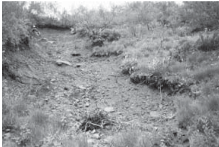
Figure 1. Medium-sized landslide in brush on basalt soils.
