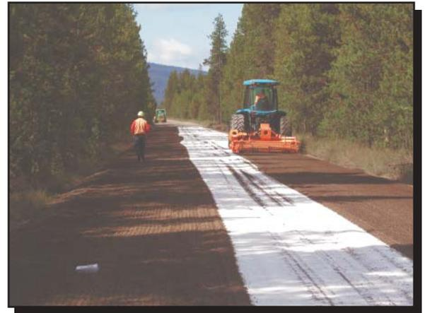
Over the next 3 years, traffic counts, weather conditions, and performance ratings will be collected for each road section. These data will be used to determine chloride's effectiveness as a stabilization agent. The test will also determine the most cost-effective and desirable form of chloride-brine (flake or pellet) and the most effective application rate and construction methods.
