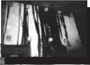
Figure 20a—Cooled asphalt dripping from the underside of the LaChance Bridge in Michigan.
