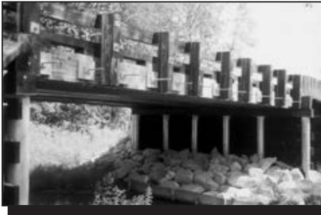
Figure 13a—The Barlow Bridge in Alcona County, MI, was made from timbers that were cleaned properly after being treated with preservative.
