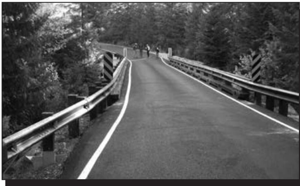
Figure 1—Paved timber bridge in Oregon.
